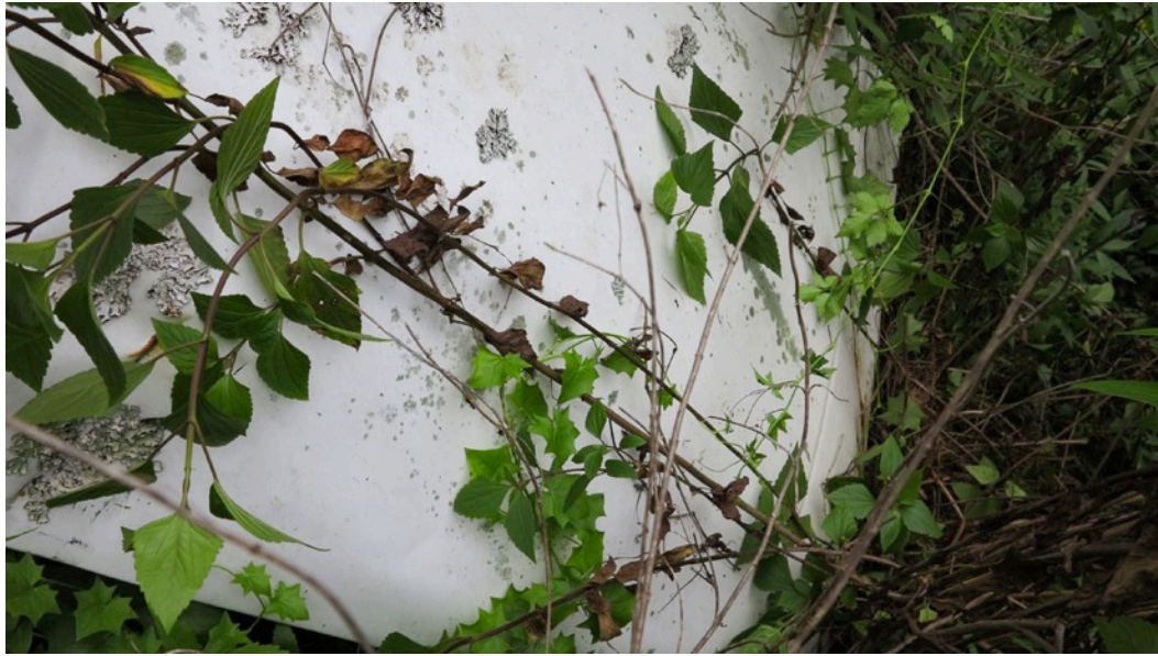
Loose bit of panel
